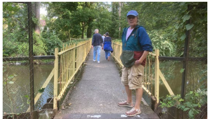
Existing Foot Bridge Across the Chadakoin River, 2023
